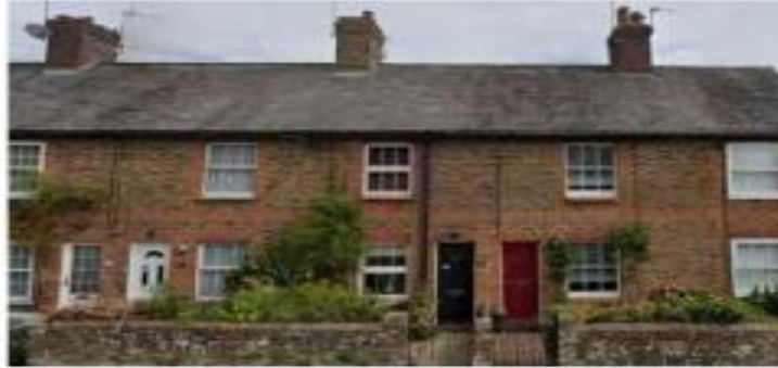
1. Terraced dwelling in brown multi-brick with red brick banding and quoining
