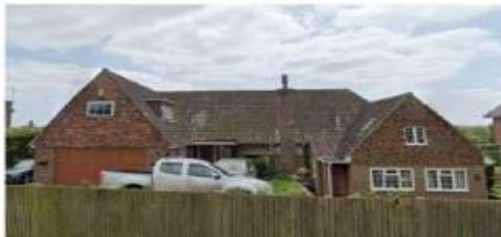
5. Detached tile hung and brick dwelling with prominent gable forms
