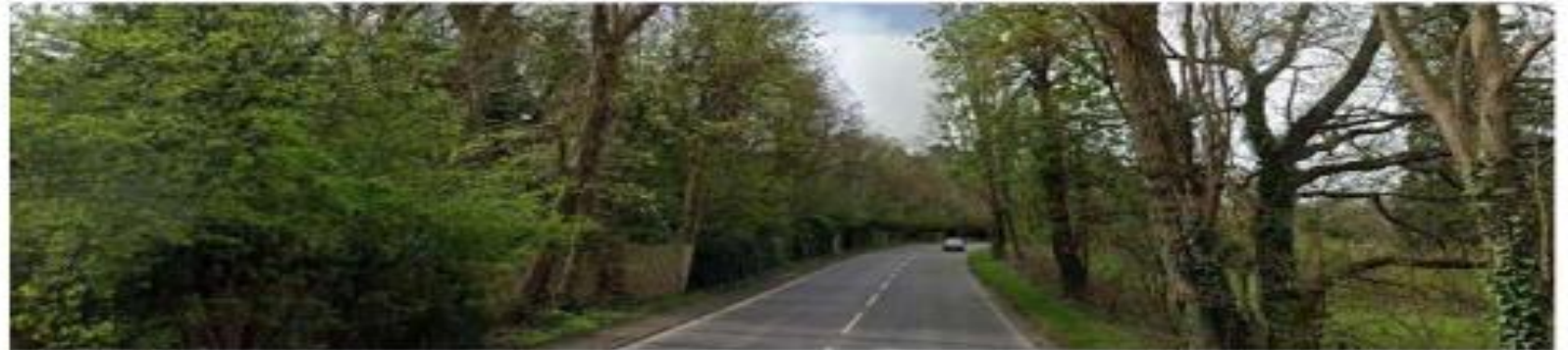
3. View looking south west along Western Road
