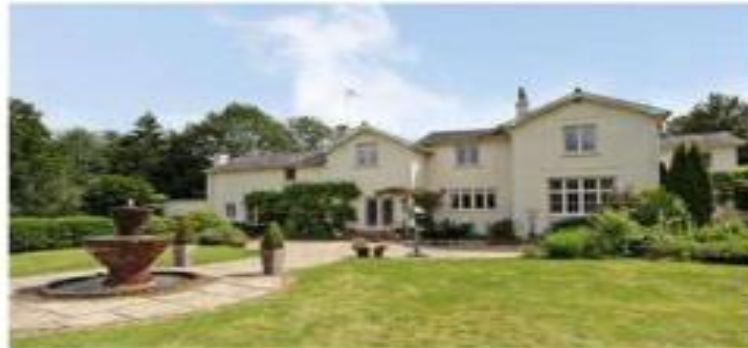
3. View looking east towards the rear elevation of Point House.
