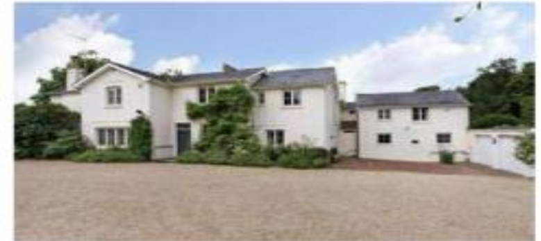
4. View looking west towards Point House from the parking forecourt.
