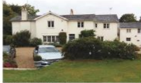
Existing Dwelling - Point House
